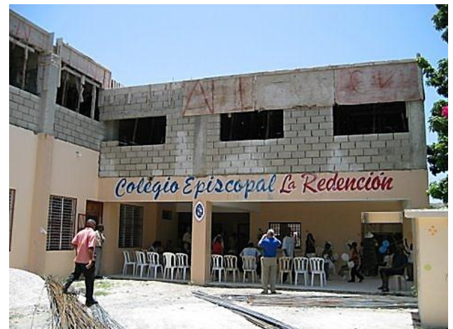
Ready to Finish: La Redención’s 2nd Floor Classrooms
